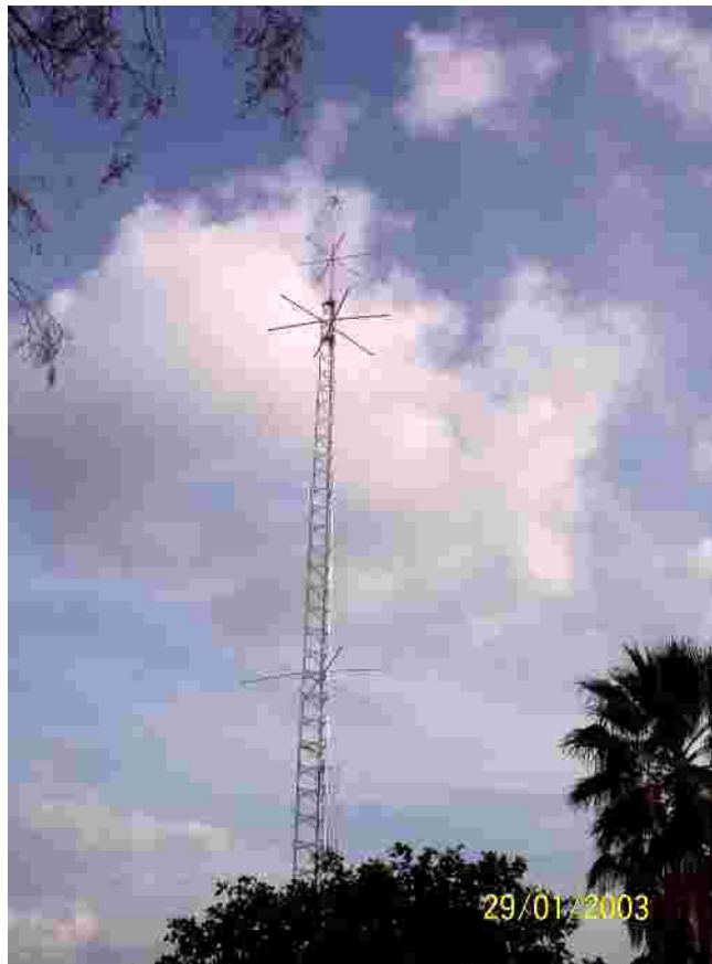
Figure 28. The pickup antenna was this 80' caged, folded monopole for the Harlingen measurements.
